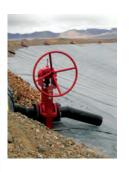
PINCH VALVES FOR THROTTLING SERVICE
